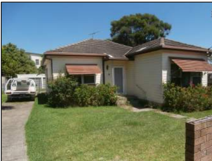
Photo 2: House on King Street to be demolished.
