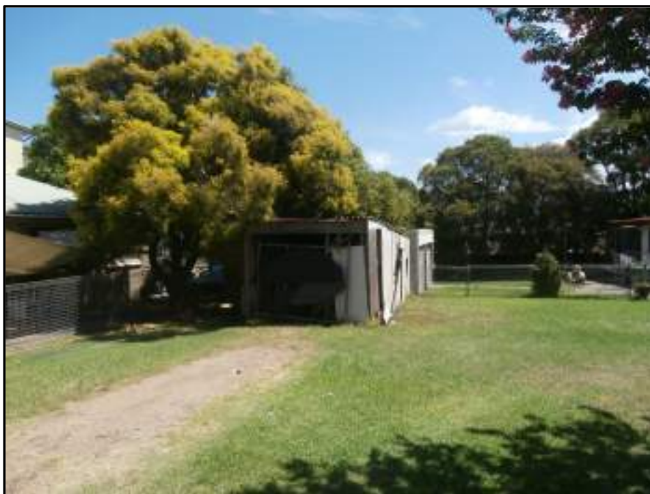
Photo 10: George and Howard Street to be demolished. Trees to be removed.
