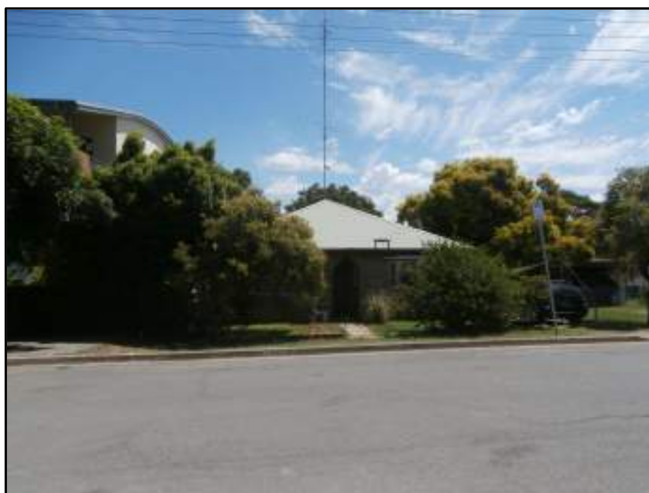
Photo 9: Dwelling on Howard Street to be demolished.
