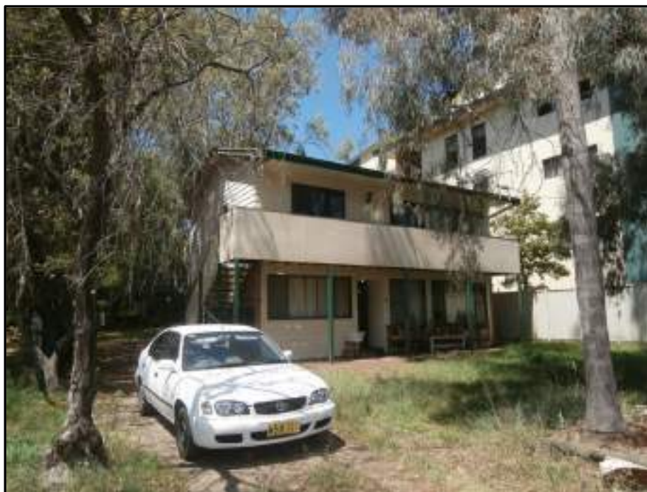
Photo 6: Dwelling on the Esplanade to be demolished.
