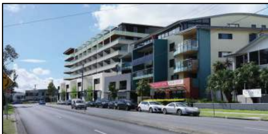
Figure 17: View from the intersection of The Esplanade and Howard Street.
